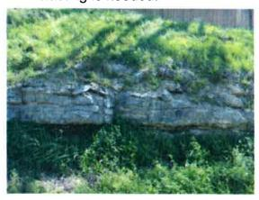
Due to the observed conditions of the masonry walls and rock cuts it is recommended that mitigation measures be undertaken and included in the proposed project. It is recommended that all unstable rock on the rock cut faces shall be trim blasted or scaled and all rockfall debris be removed from inside the catchment area behind the rockfall fences.
